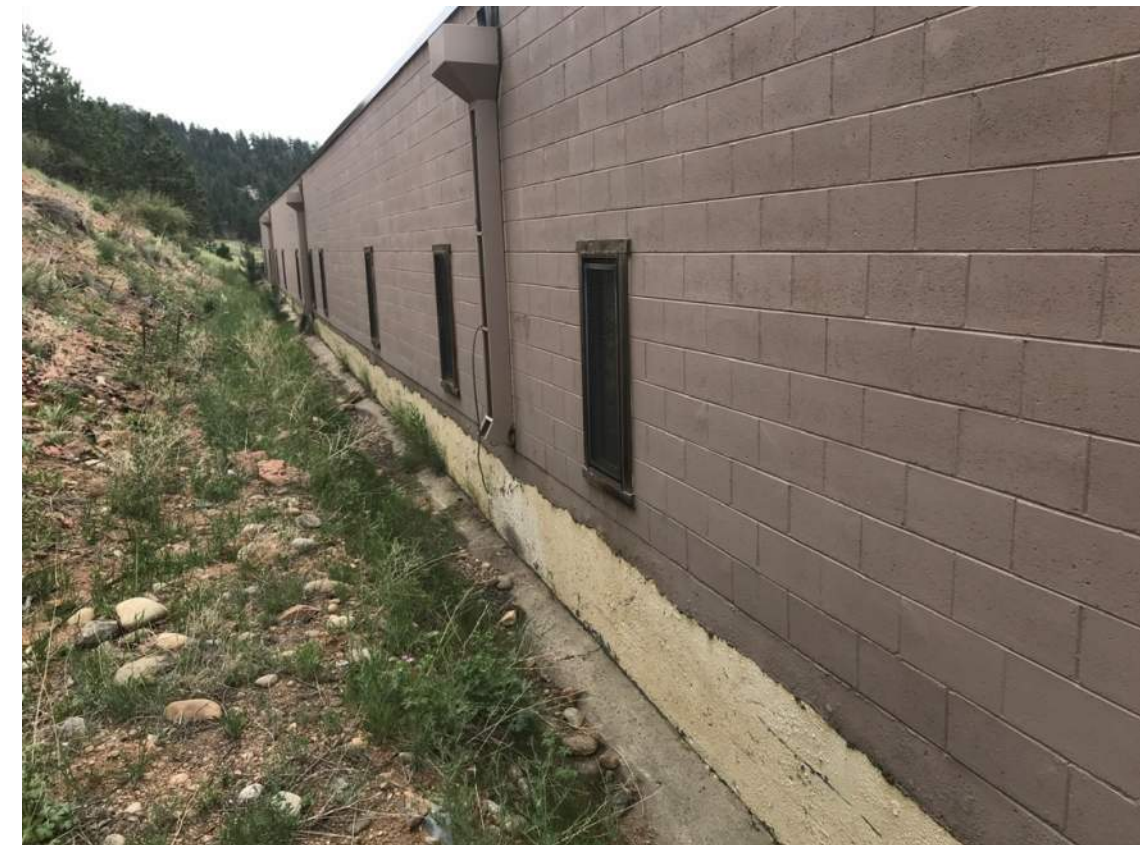
NORTH SIDE DRAINAGE ISSUES
