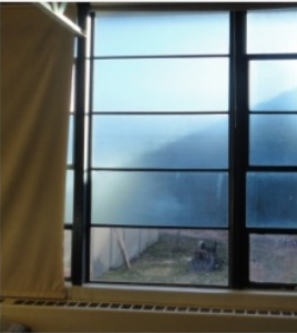
Failing, energy inefficient single glazing
