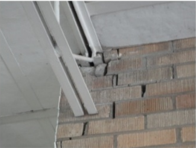
Cracking masonry at structural connection
