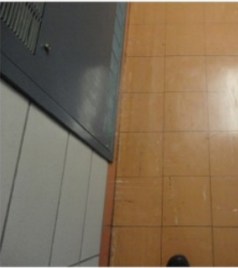
Asbestos floor tile
