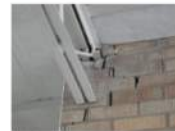
Cracking masonry at structural connection
