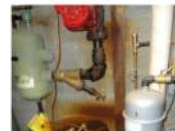
Antique, aging water system
