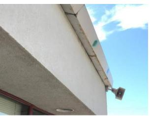
Replace leaking gutter. Possible soffit damage
