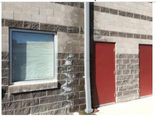
Repair leaking gutters causing an ice hazard
