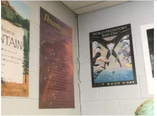
Settlement cracks in interior CMU walls
