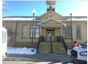
Replace front entry stairs that are deteiorating from freeze and thaw
