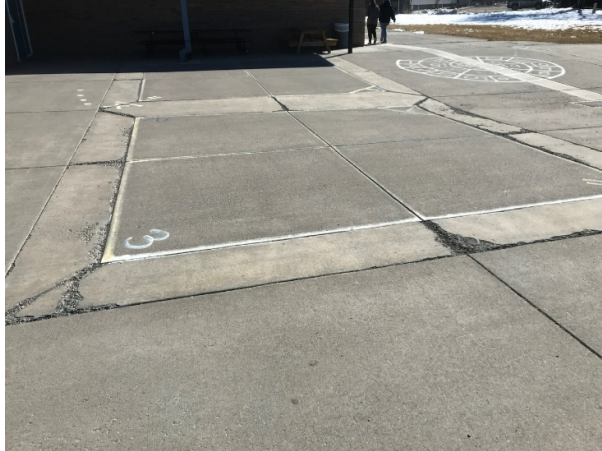
Replace sinking/uplifting side walks
