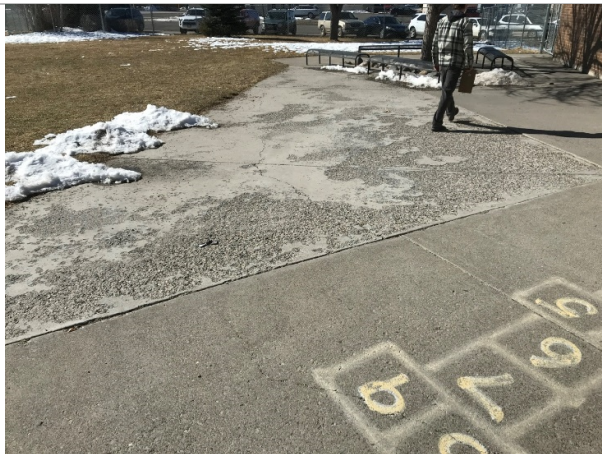
Repair settled concrete side walk
