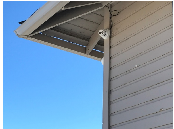
Replace rotting eaves
