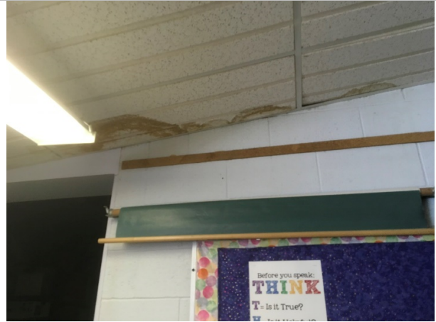
Roof leak in 302
