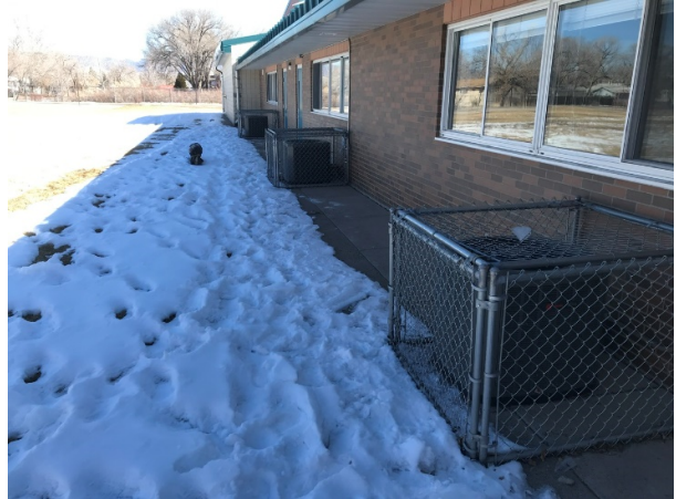
Provide snow stops at critical areas
