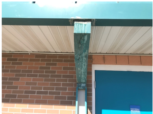
Correct/replace down spouts/gutters
