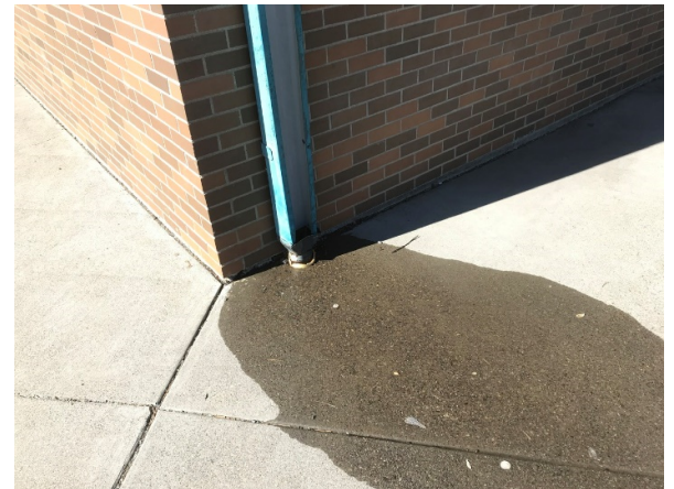
Replace downspouts that are deteriorating and causing an ice hazard
