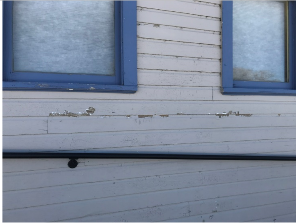
Replace deteriorated wood siding
