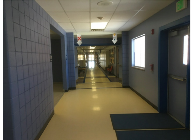
Corridor 101 – walls not to doc, doors, and frames not fire rated
