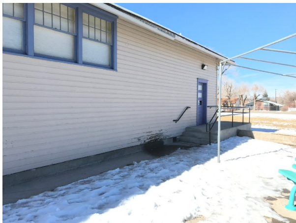
Provide snow guards on roof at exterior doors
