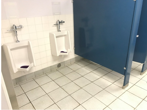
Provide urinal screens
