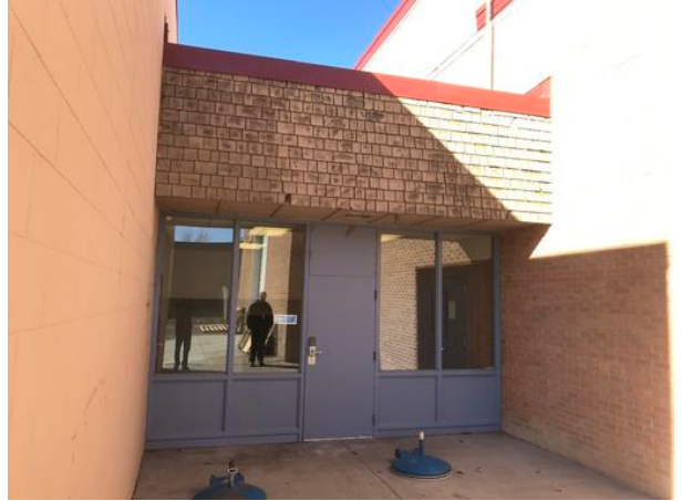
Replace single pane windows in south building
