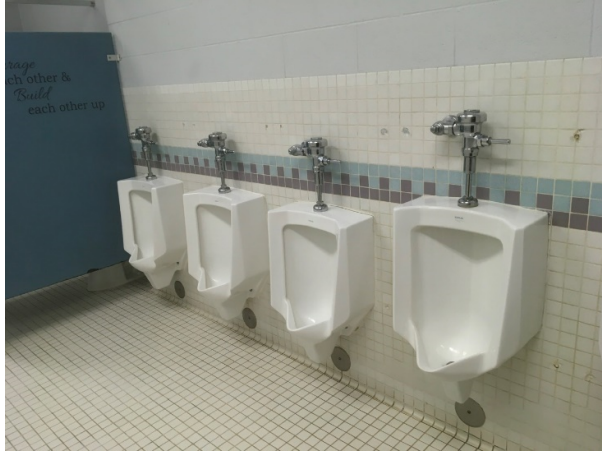
Lack of screening in main restrooms
