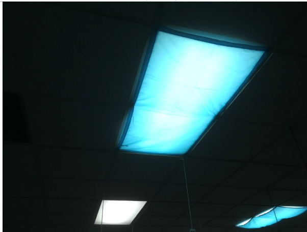
Flourescent lighting cover due to undesirable light output
