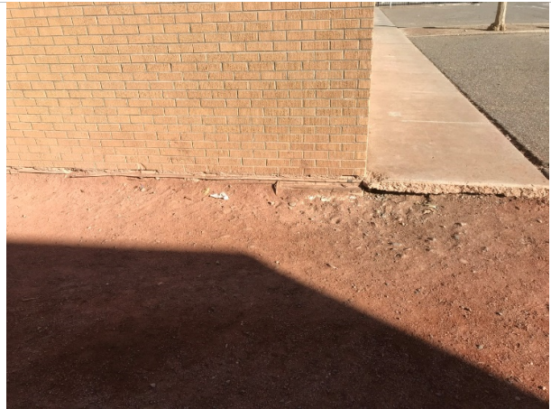
Broken sidewalk and deteriorated brick
