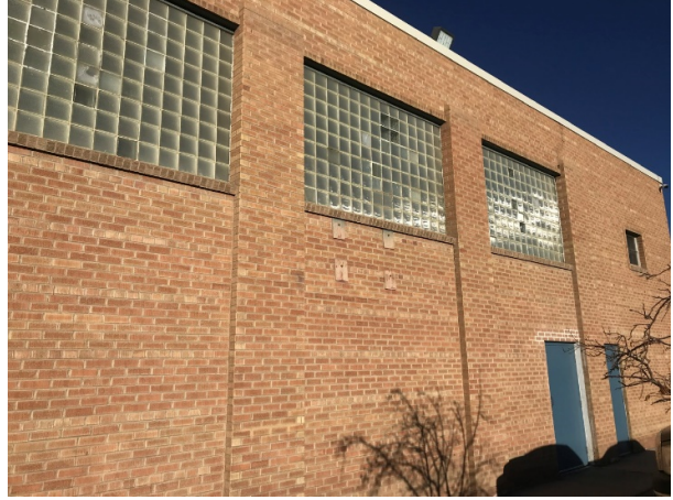
Inefficient glass block openings
