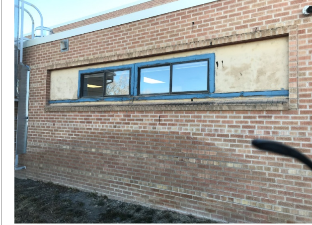
Deteriorated wood at exterior windows
