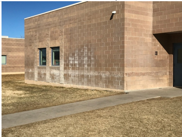
Effervescent on exterior wall
