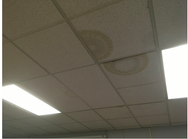
Water damage in interior ceiling tiles
