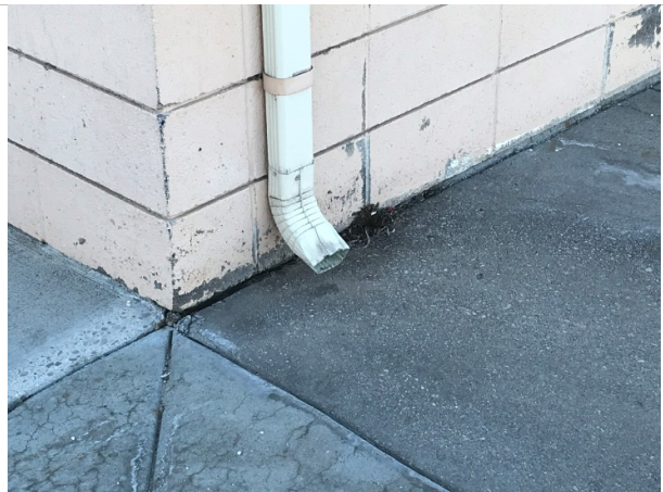
Downspout at sidewalk / icing issues
