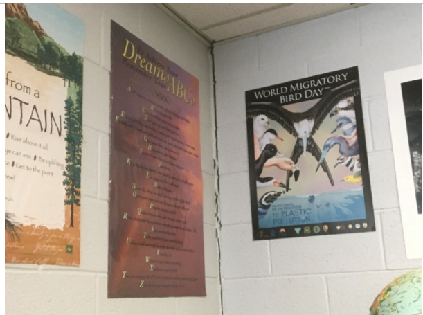
Settlement cracks in interior CMU walls
