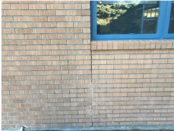
Deteriorated caulk joints
