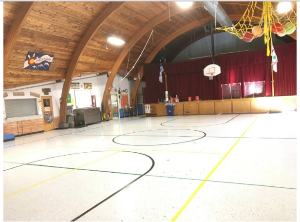
Provide ADA access to stage
