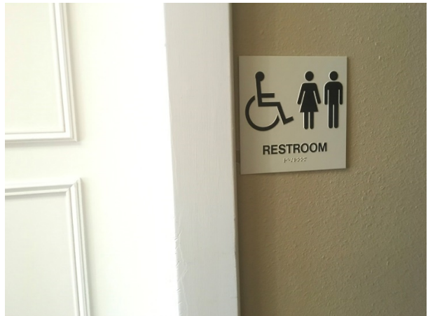
Provide ADA compliant door signage
