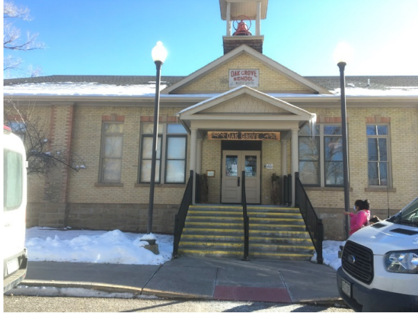
Replace front entry stairs that are deteriorating from freeze and thaw
