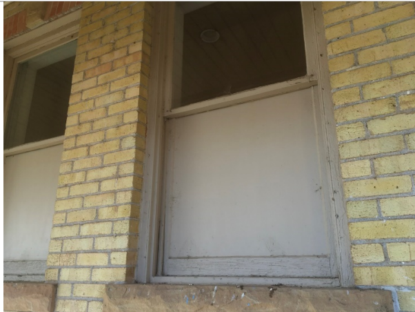
Replace windows in bathroom, library, 400 wing, and original building
