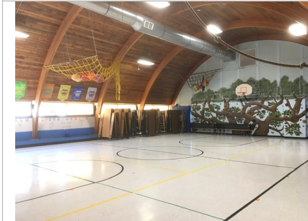
Replace rotten wood on multi-colored wall at north of gym
