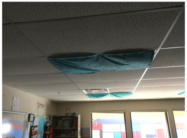
Replace deteriorates ceiling tiles
