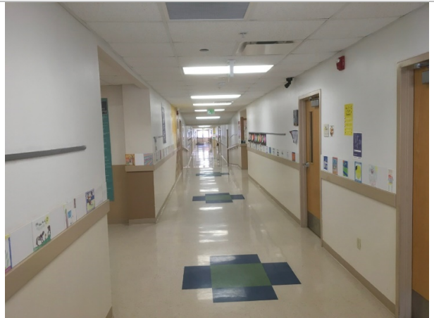
The corridors and classrooms have fluorescent lighting
