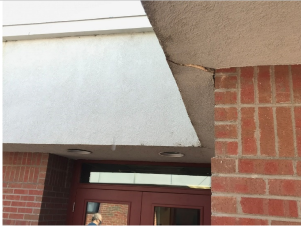
Caulking needs to be redone around windows and control joints
