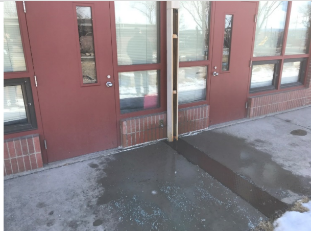
Roof dripping on sidewalk in front of classroom doors
