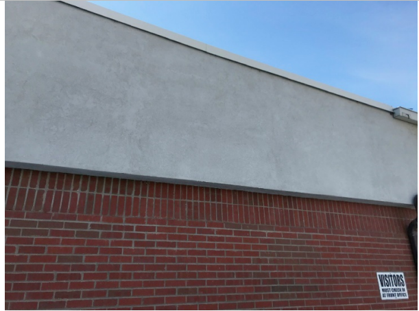
Provide missing roof gutters
