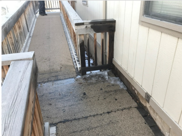
Wooden ramp back of building has roof drain leaking
