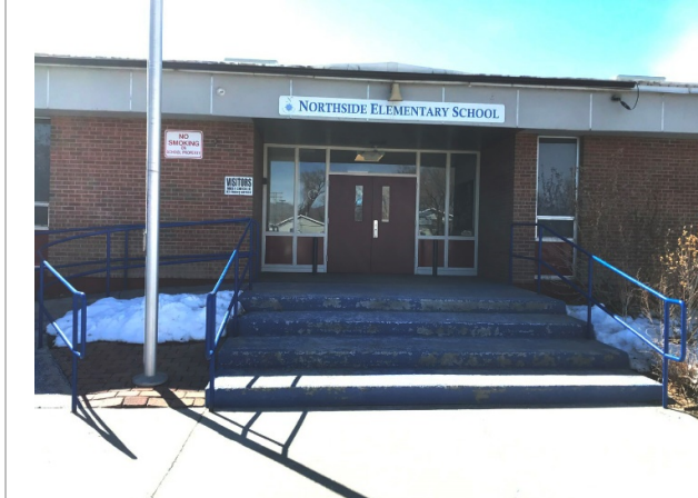
Replace single pane wire glass at main entry
