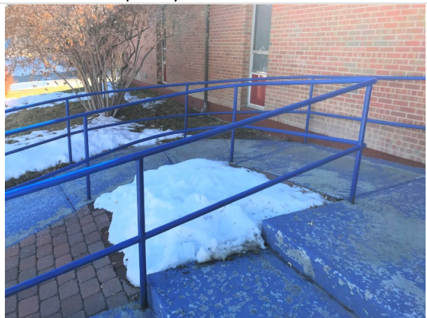
Handicap ramp does not meet ADA requirements
