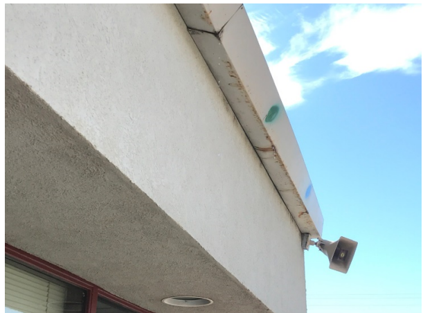
Replace leaking gutter. Possible soffit damage
