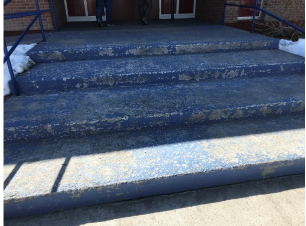
Main sidewalk concrete is deteriorated and is hazardous
