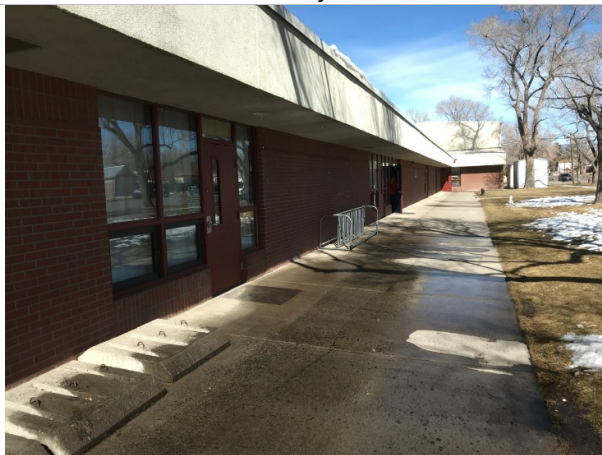
Replace single pane window in old building
