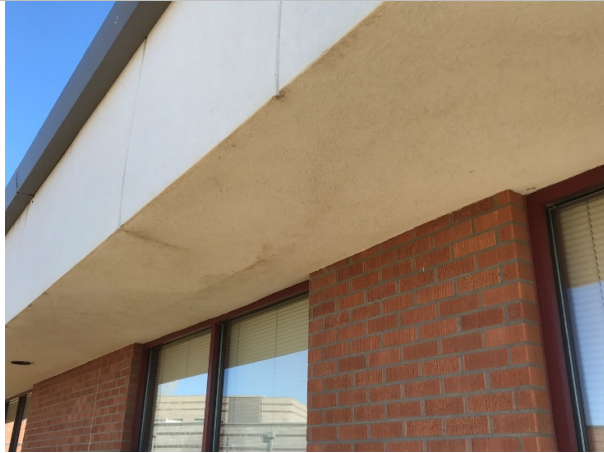
Replace leaking gutters
