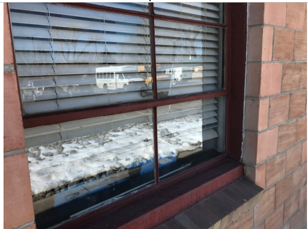
Replace caulking around expansion joints and windows
