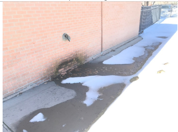
Correct east lamb's tongue that is dripping onto the sidewalk
