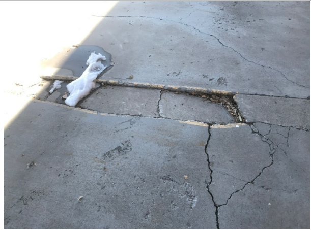
Replace sidewalks that are sagging 4" +/- and causing safety issues
