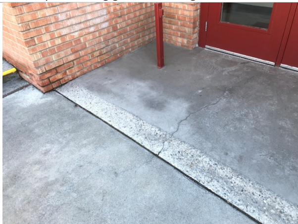
Replace concrete because of water ponding at entry
