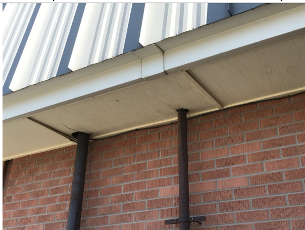
Replace seperating soffit plywood
