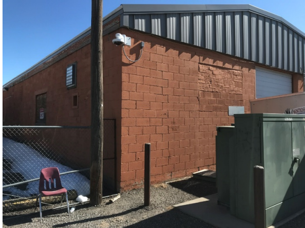
Provide gutters on shed roofs, dumping ewater onto main walkway
