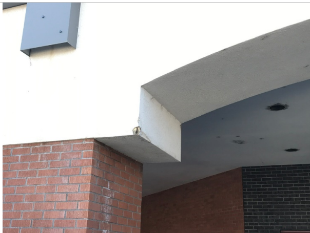
Replace the stucco southwest of main entry
