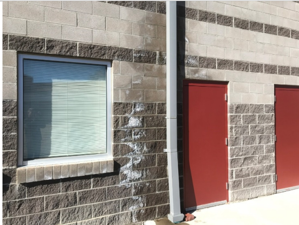
Repair leaking gutters causing an ice hazard
