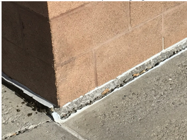
Replace Caulking at site hardscapes
