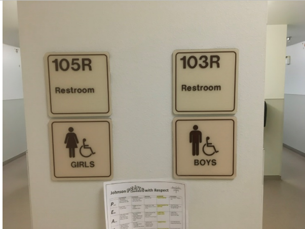
Provide ADA compliant signage
