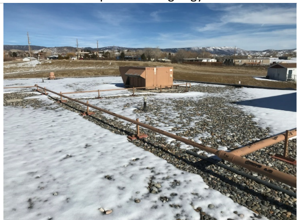
Out of date rooftop mechanical systems
