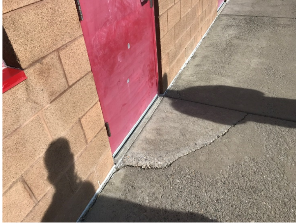
Replace displaced sidewalk
