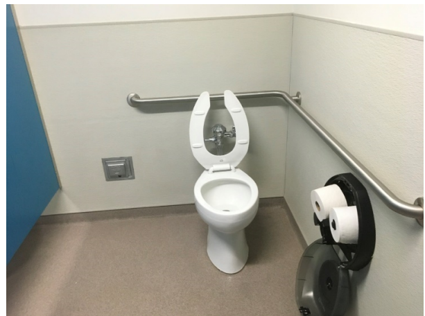
Replace continual grab bars with segmented ones
