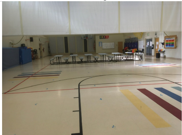
Replace flooring in gym
