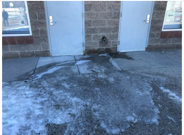
Redirect water from the lambs tongue between two doors causing an ice hazard
