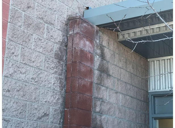
Provide a gutter at north entrance due to icy buildup
