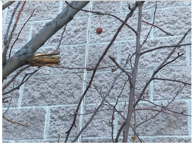
Seal masonry at northwest elevation
