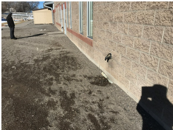
Redirect water from the lambs tongue on south side of the building
