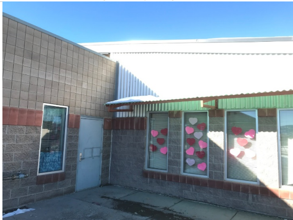
Repair loose overhang and gutter that has failed and causing an ice hazard
