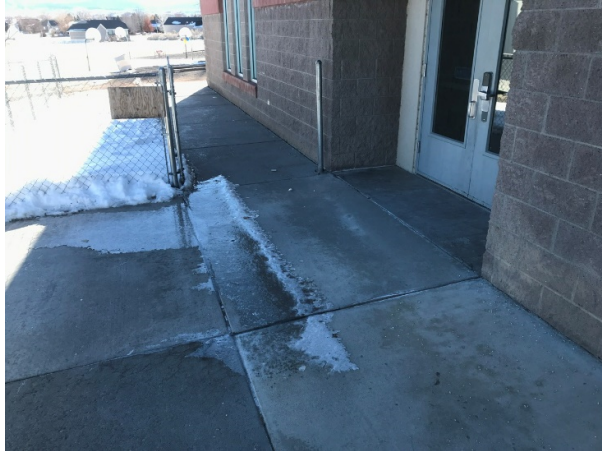
Redirect a gutter spilling onto sidewalk
