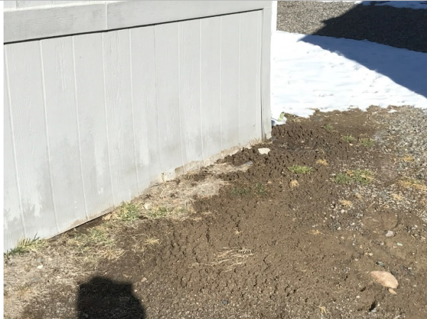
Grade at some points are high and rotting the plywood skirt
