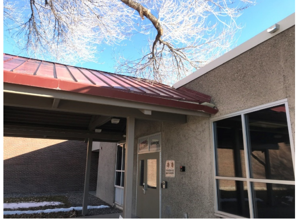
Replace damaged gutter
