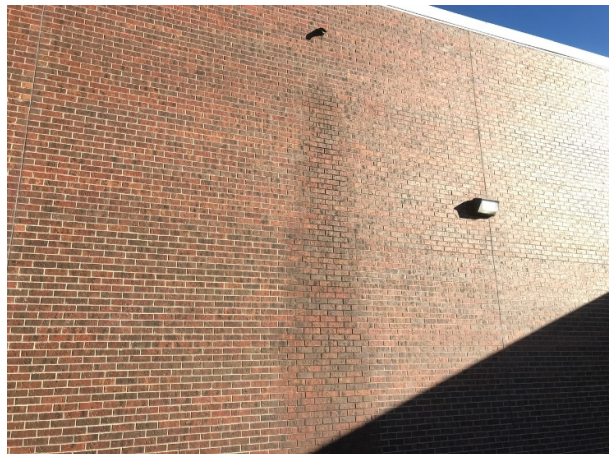
Downspout off of gym leaks on face of brick
