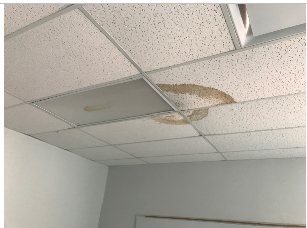
Replace ceiling tiles that are outdated
