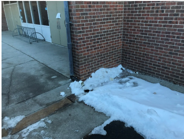
Reroute downspout at the north entry that cases ice hazards
