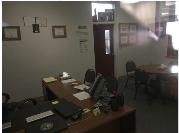
South side door in principal's office has non-compliant door hardware
