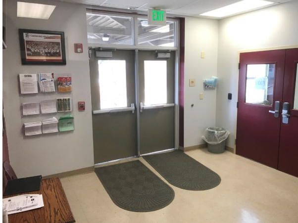
Replace wire glass on exterior door
