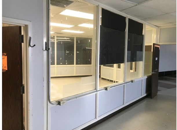
Replace single pane wired glass all locations
