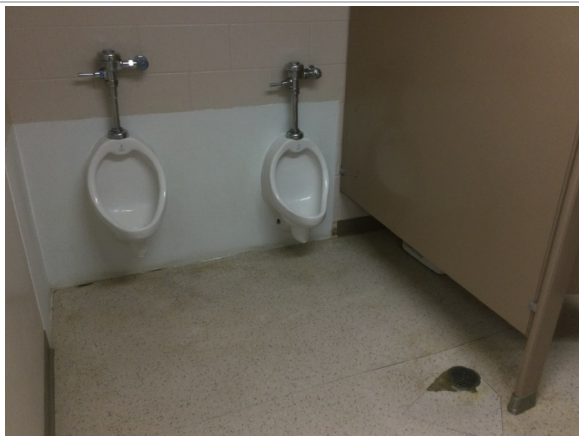
Replace restroom flooring
