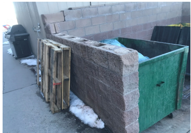
Repair CMU wall and provide cap stones
