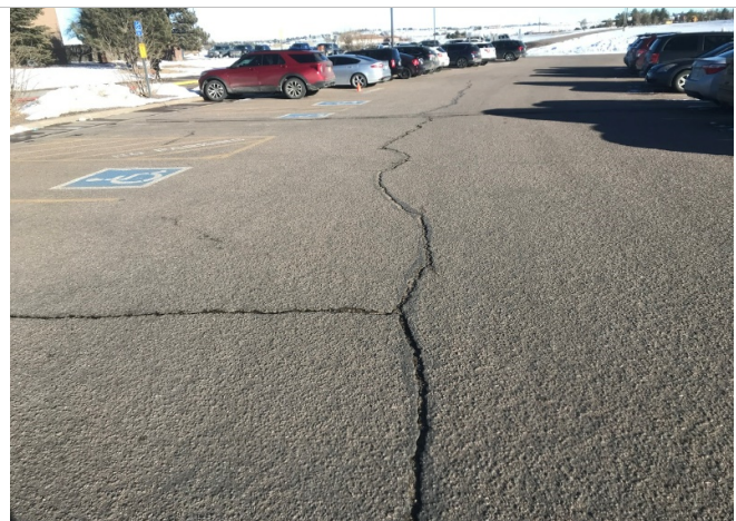
Repair cracks throughout parking lot
