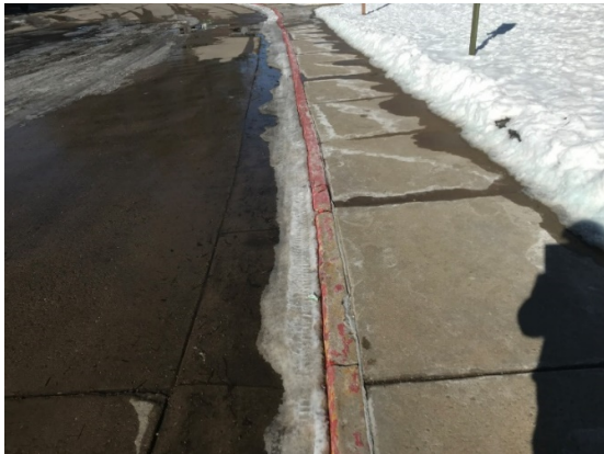
Replace curb and gutter
