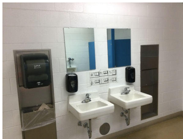
Provide pipe wrap at sinks
