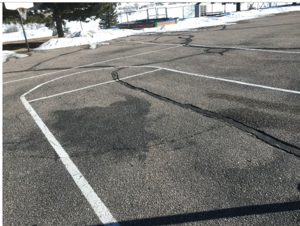
Repair asphalt at playground
