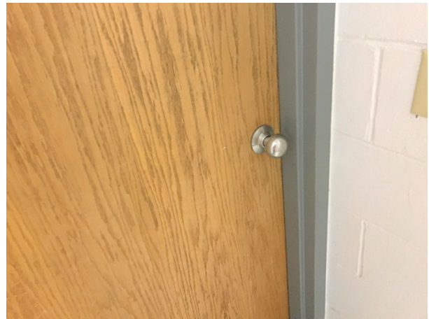
Provide ADA-compliant door hardware
