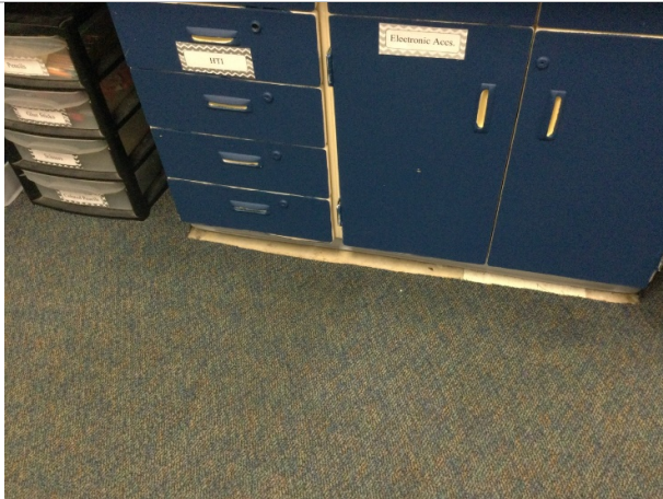
Replace classroom flooring
