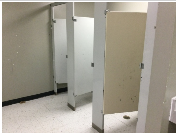
Replace restroom partitions
