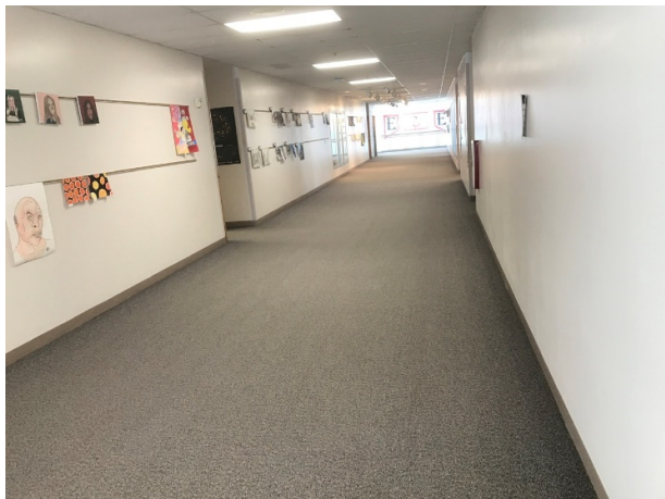
Replace classroom and corridor flooring
