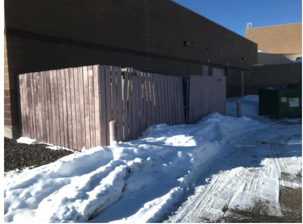
Replace fence around utilities
