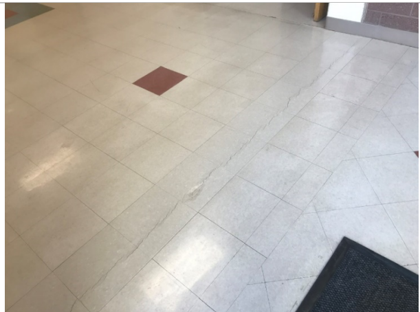
Replace cafeteria flooring
