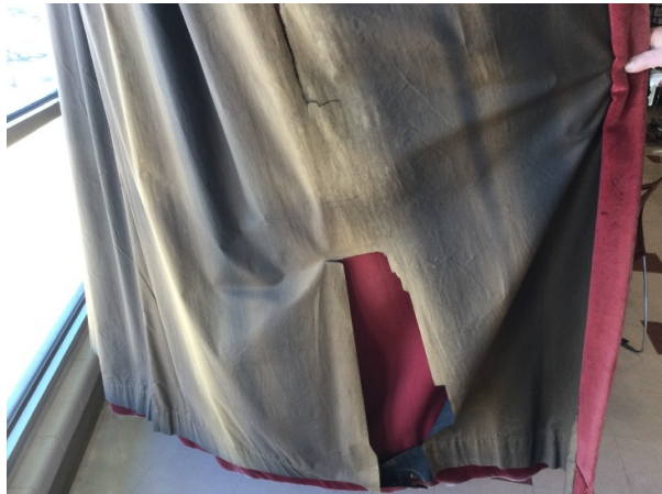
Replace window covering at cafeteria
