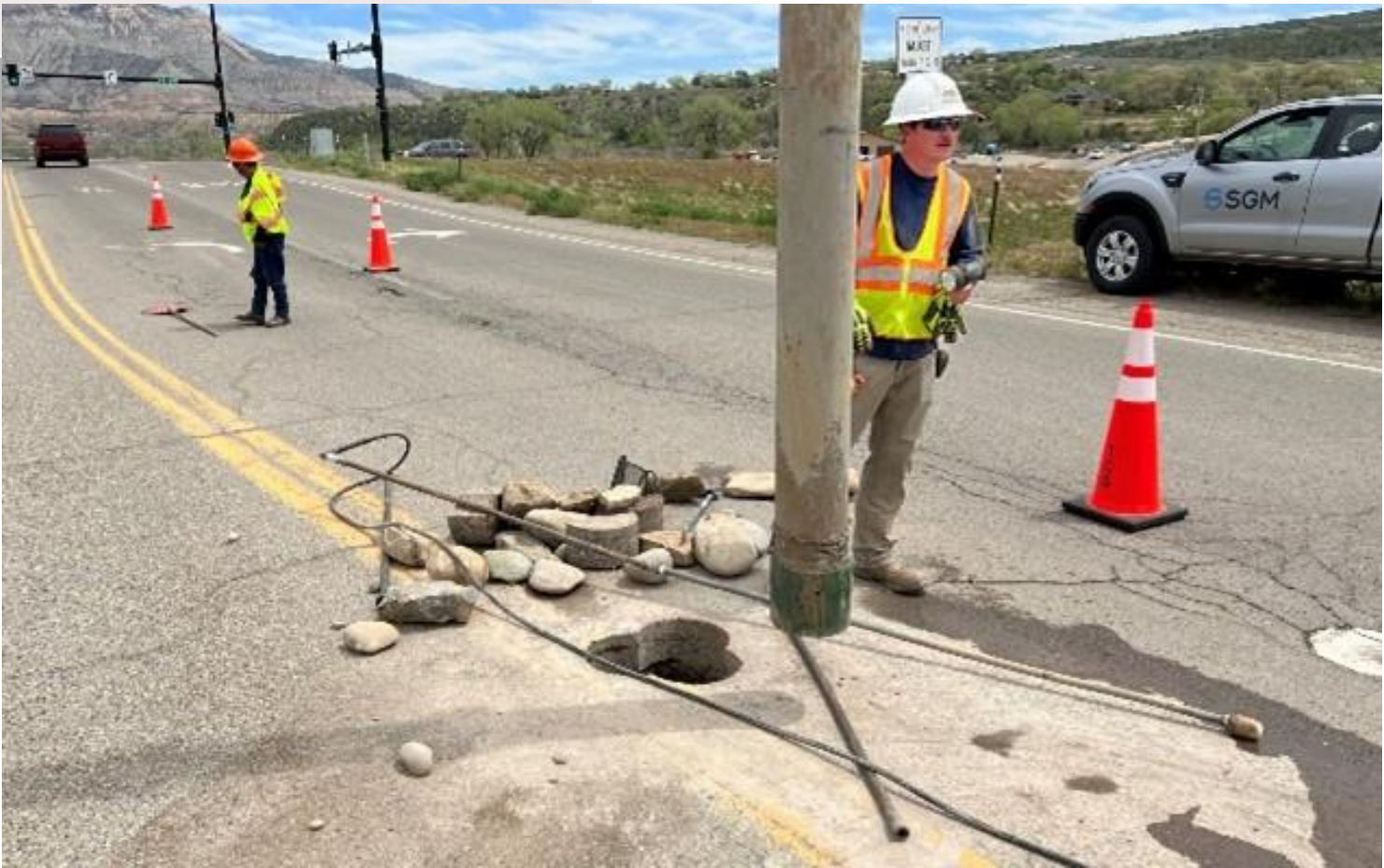
Test hole exploration for utility work – Grand Junction, CO
