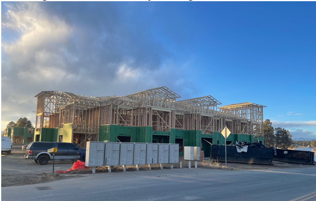
Figure 8 - New Multi-family Housing Under Construction
