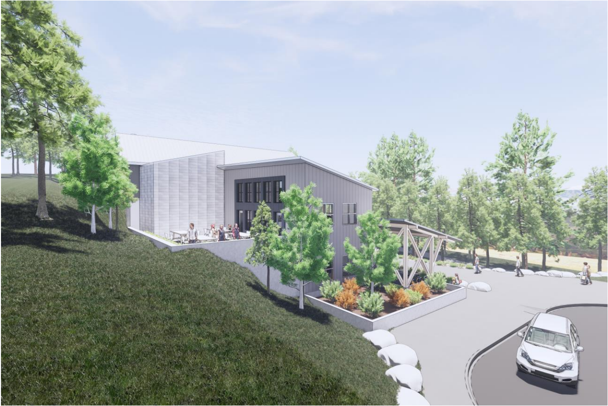
Phase 1 Addition – from Society Drive looking northwest
